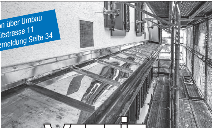
Renovation Restaurant Sonnenhof
